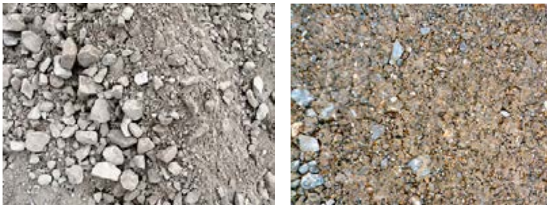
Figure 12 & 13 - Loose / Compacted base material
