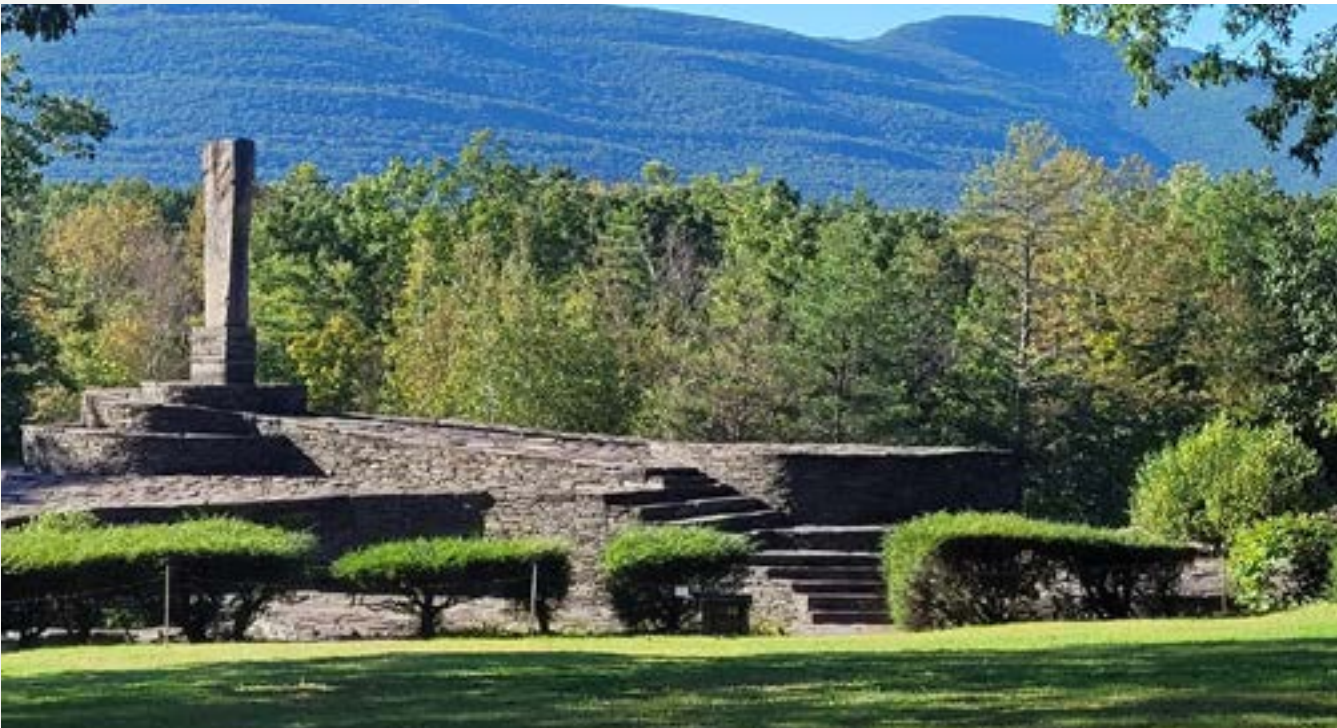
Figure 27 -Natural stone wall
